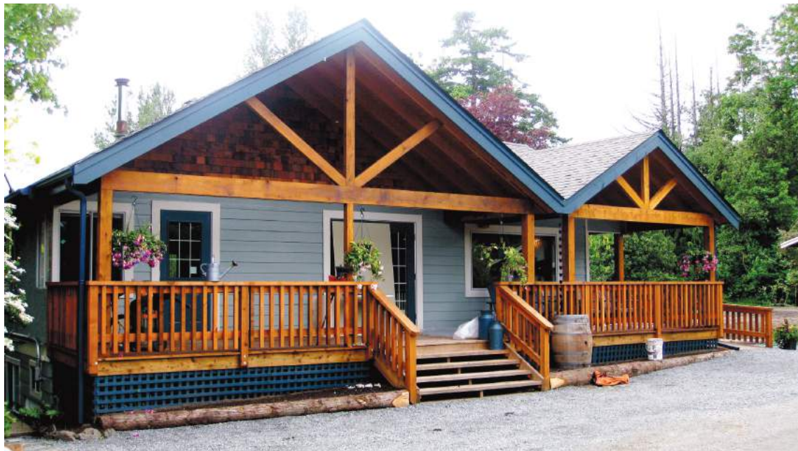
Sargent Construction specializes in new construction and renovations such as this Chemainus Garden Expo office reno
